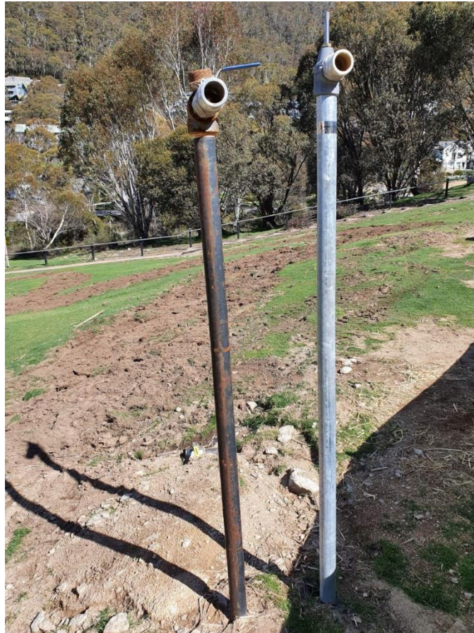
Figure 5: Example of a manual hydrant
